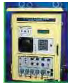
Underwater Telephone System
