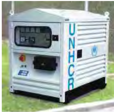
Diesel Generating Set
