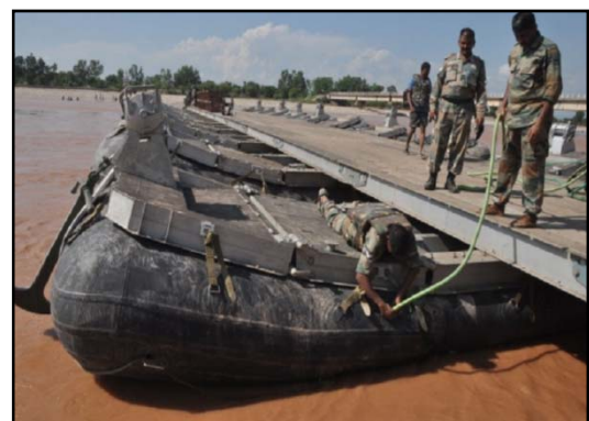
JAMMU, INDIA - 2014/09/09: A soldier of Indian Army's engineer core pumps air into inflatable tubes as they build a pontoon bridge across river Tawi in Mandal area of Jammu. (Photo by Pacific Press/LightRocket via Getty Images)
