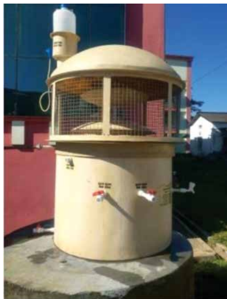
Iron Removal Unit (300 l/hr)
