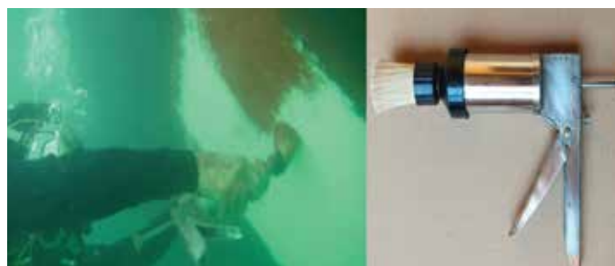
Diver applying underwater paint
