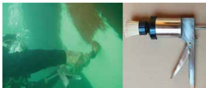
Diver applying underwater paint
