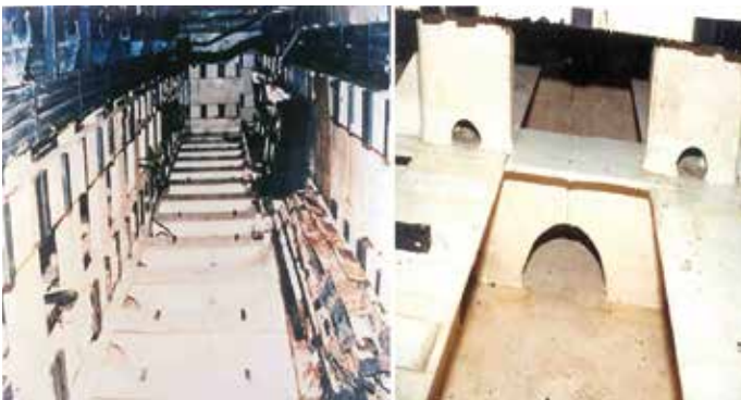
Solvent-free anti-corrosive paint applied in battery pit of submarine
