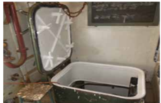
Engine room hatch area of ship coated with self-cleaning coating
