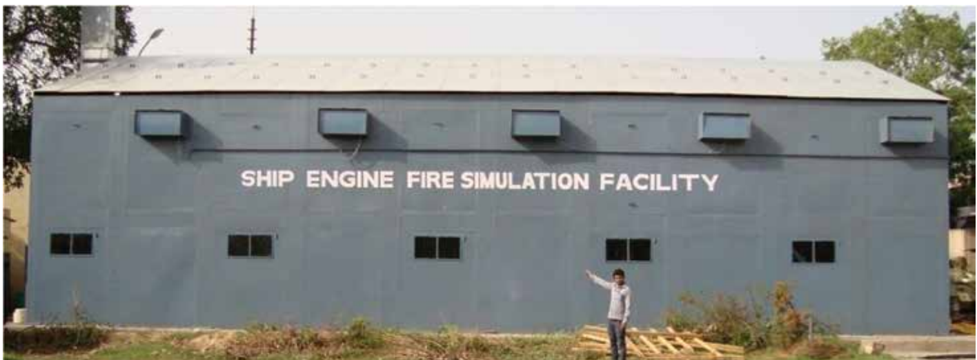
1000 m 3 engine fire simulation facility
