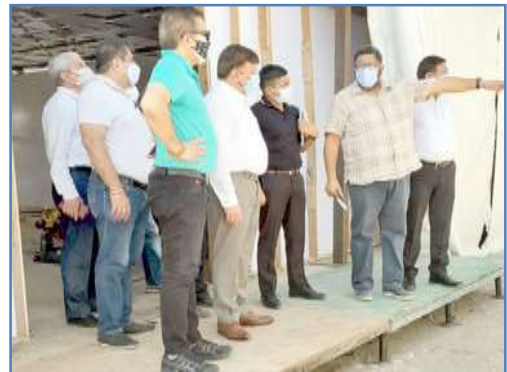
CCI team visiting under construction COVID hospital at Bhagwati Nagar, Jammu on Saturday.
