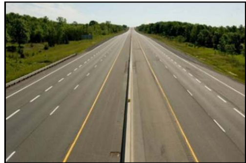
An MoU was signed between the Road Transport and Highways Ministry and DRDO on January 20.
