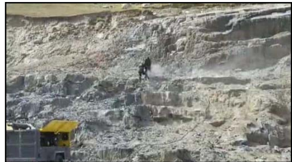
Photo of blasting process for Zojila tunnel construction. (Hindustan Times)
