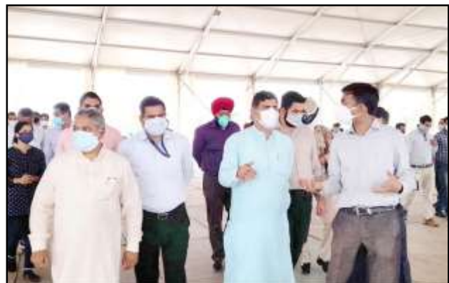
MP, Jugal Kishore Sharma inspecting under construction DRDO Hospital at Jammu on Thursday.
