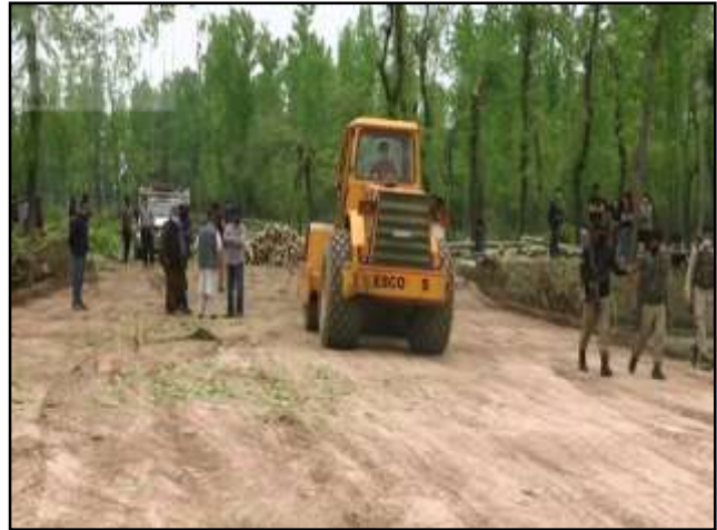
DRDO starts construction of 500-bed COVID-19 hospital in J-K's Budgam (Photo/ANI)
