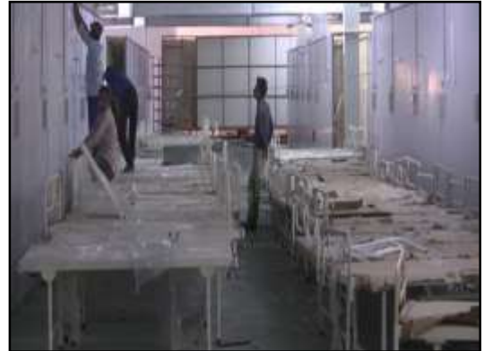
J-K: Srinagar's 500 bed Covid-19 hospital in final stages of completion
