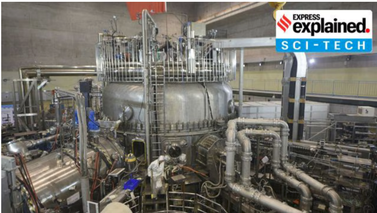
Experimental Advanced Superconducting Tokamak (EAST), a nuclear fusion reactor, in Hefei, Anhui province, China
