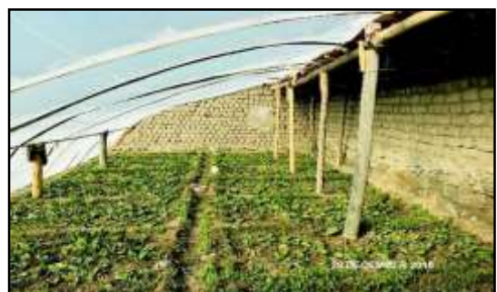
The older iteration of the passive solar greenhouse
