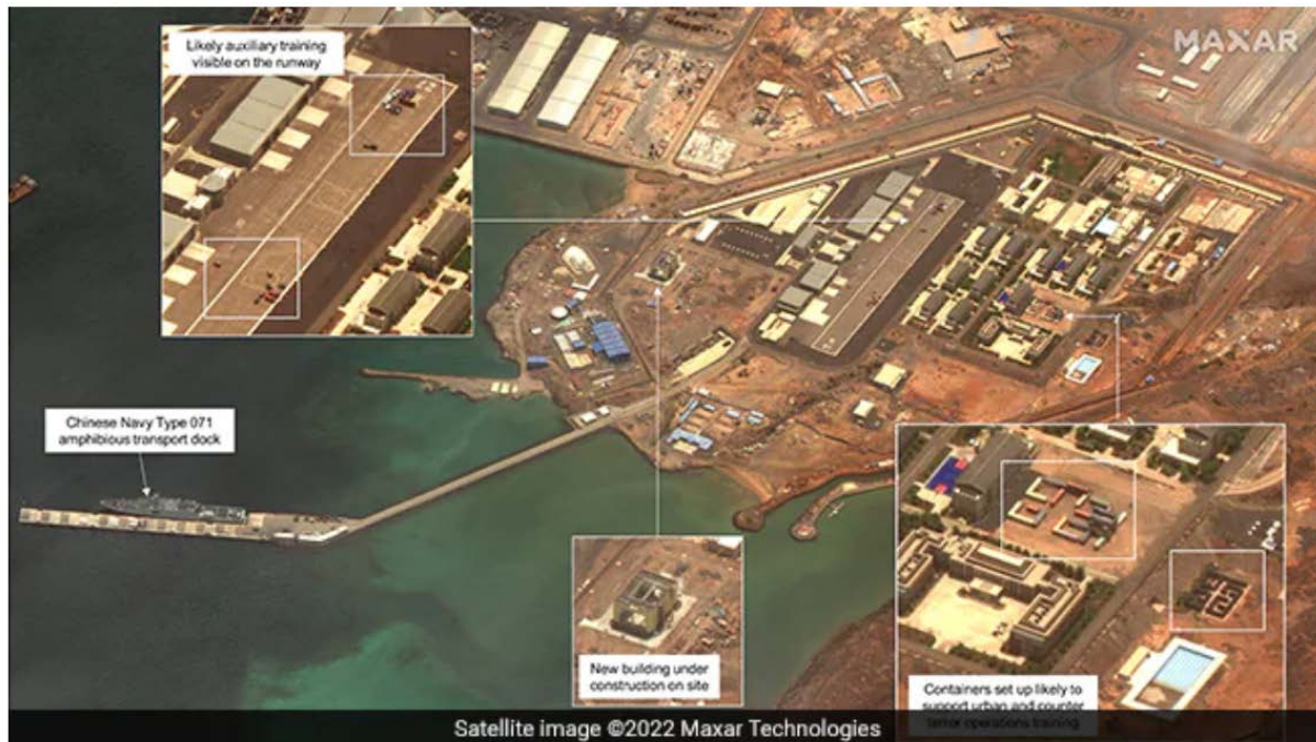
Chinese naval base in Djibouti, fully operational. With inputs Damien Symon. High-res here
