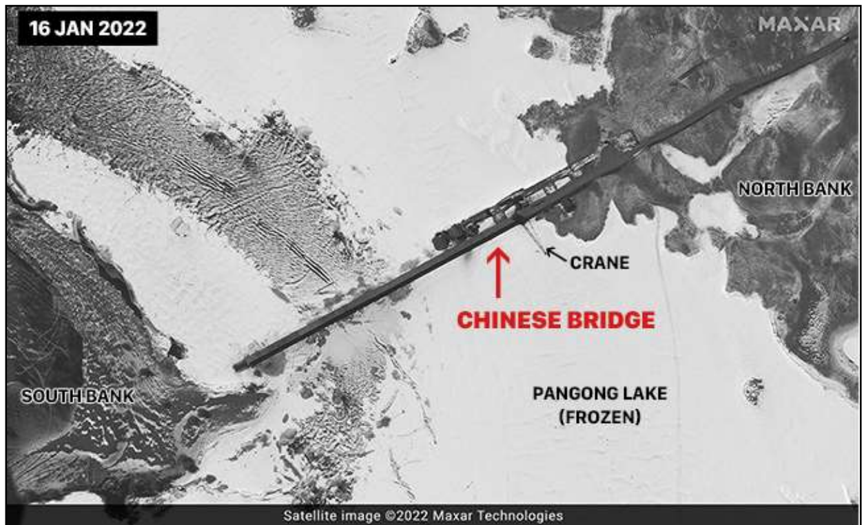
China's illegal bridge across a frozen Pangong Lake is seen being constructed with a heavy crane in satellite images. High-res here
