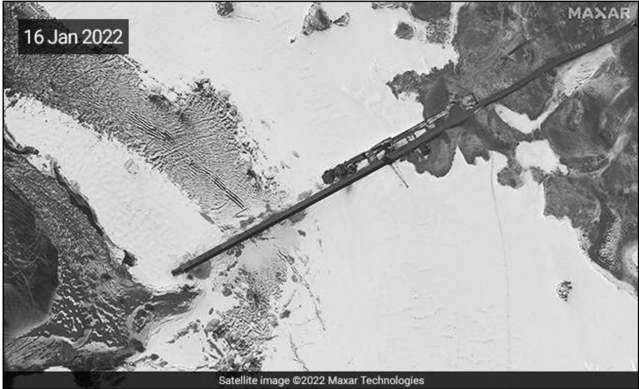
China's bridge across frozen Pangong Lake will link roads on North and South Banks. High-res here
