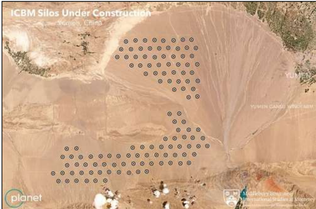
Images of Yumen Silo Field, where China may be constructing 120 missile silos. (Credit: Planet Labs Inc)
