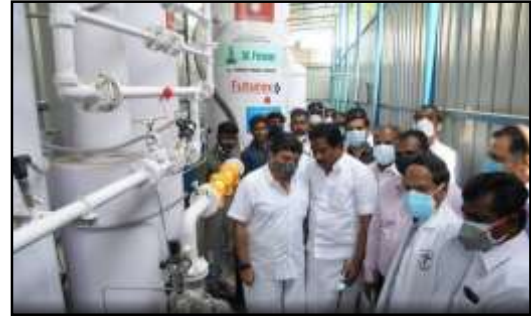
A new oxygen generator donated by philanthropists was commissioned at Government Rajaji Hospital in Madurai on Sunday. | Photo Credit: G. Moorthy
