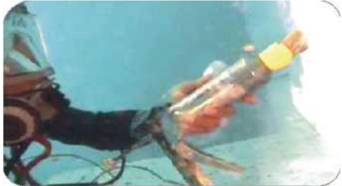
In situ underwater painting on ship hull
