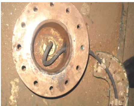
Surface preparation of cofferdam
