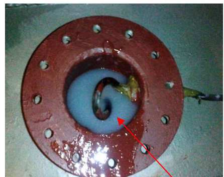
Cofferdam filled with potting material
