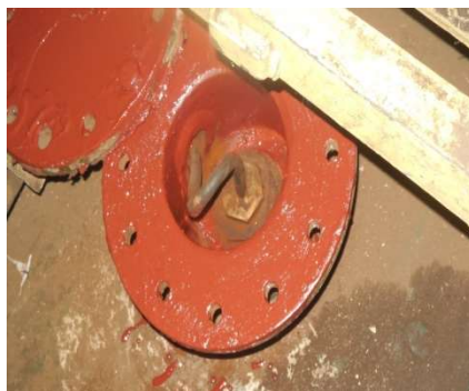
Cofferdam coated with primer
