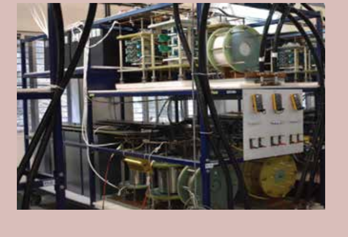
CAD Model and Realized Capacitor Bank Module Arranged on a Rack
