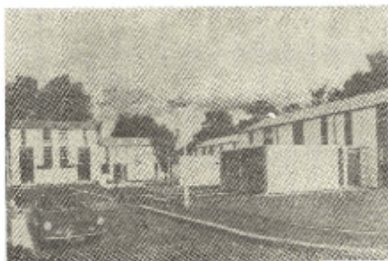
Fig. 28 Three-storeyed dwellings constructed from GRP load-bearing panels
