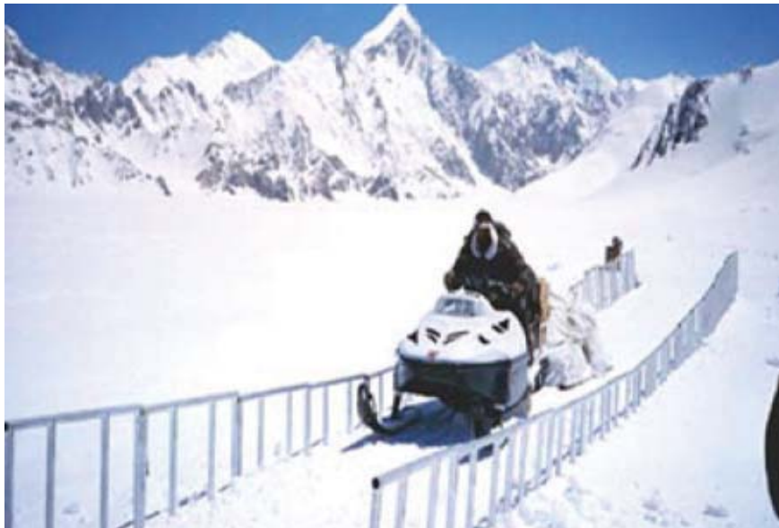
Crevasse Crossing Bridge
