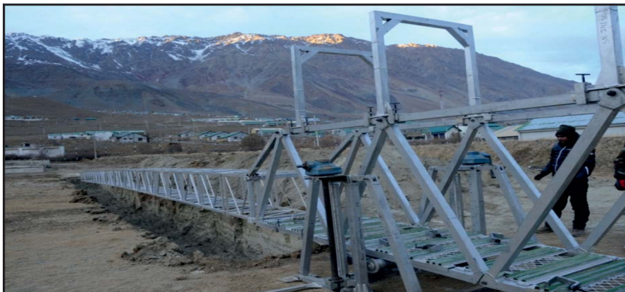
35 m Mountain Foot Bridge
